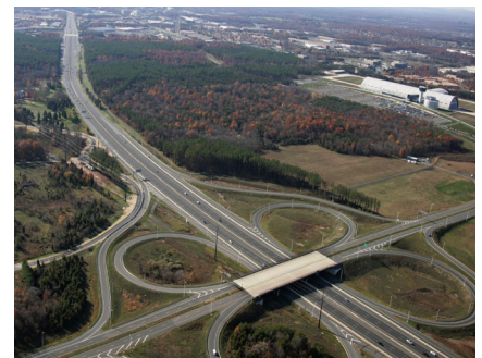
Route 28 Corridor Improvements Project for Fairfax and Loudoun Counties was constructed by Shirley and designed by Dewberry. The project converted 10 intersections to grade separated intersection and included secondary road improvements.
