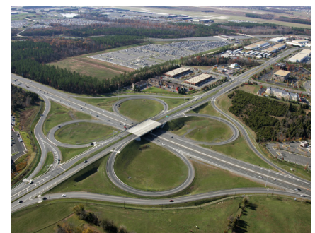
Dewberry is the Lead Designer on the Route 28 Corridor Improvements with Shirley, pictured above is Route 28 at Route 606 in Loudoun County, Virginia.
