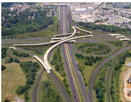
The $513 million design-build Contract C of the Intercounty Connector calls for the design and construction of a nearly four-mile long, six-lane segment of the ICC from west of US 29 to east of I-95.
